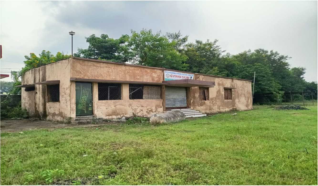
Multi Utility Hall
